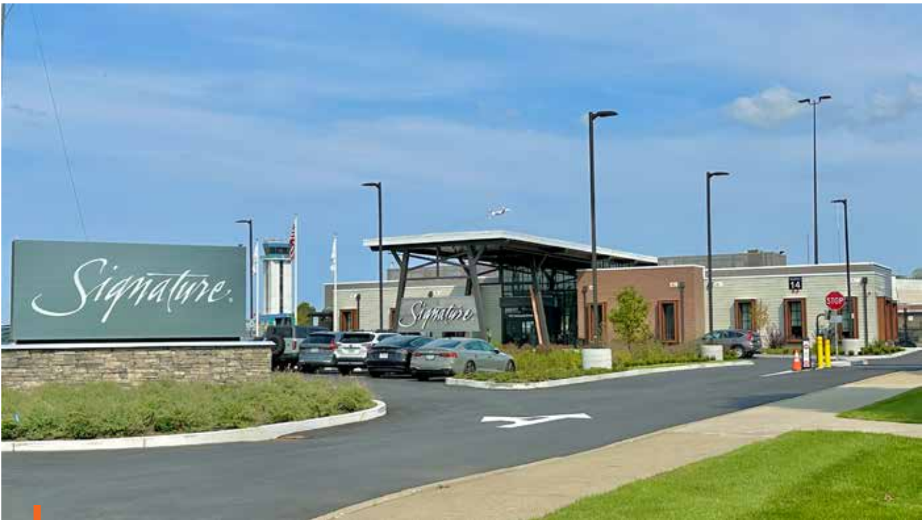
Signature Aviation's new facility at Hanscom opened in 2023.
