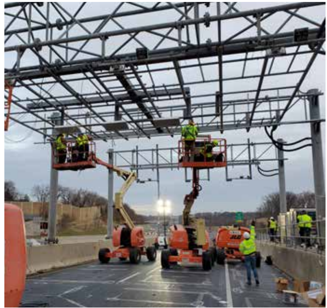
I-95 Express Toll Lanes gantries.
