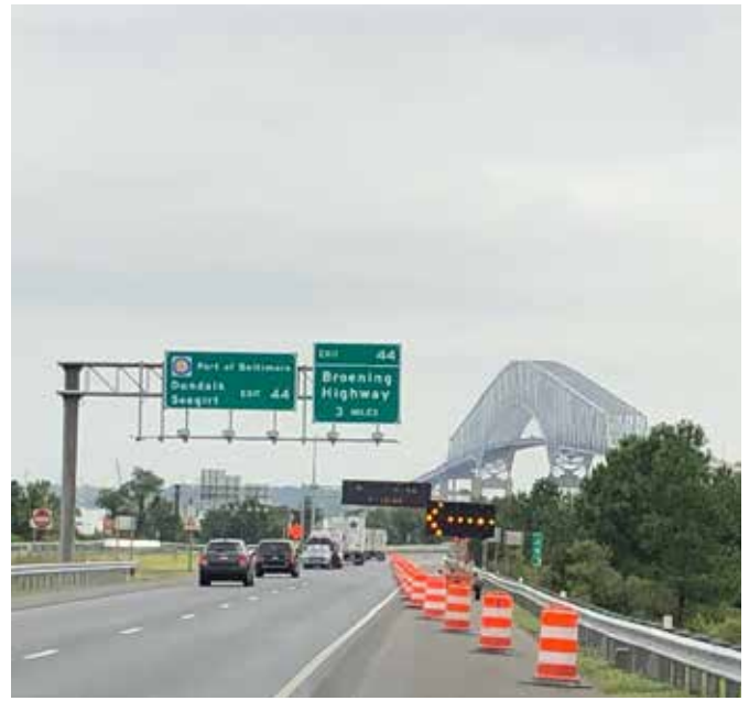
Maintenance of Traffic devices at the Key Bridge.
