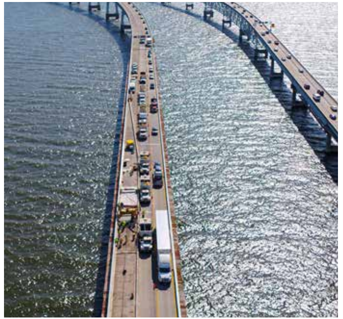
Bay Bridge Westbound Rehabilitation Project
