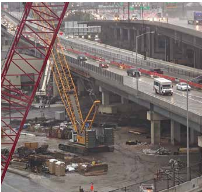
I-895 Bridge Project
