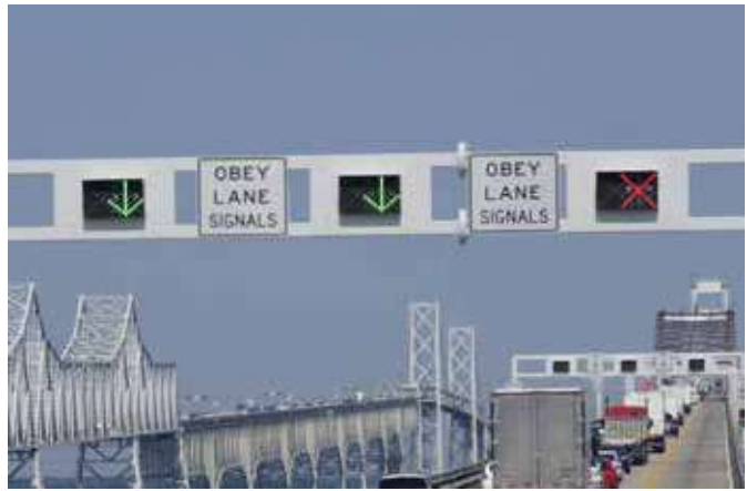
Overhead Lane Use Signals at the Bay Bridge
