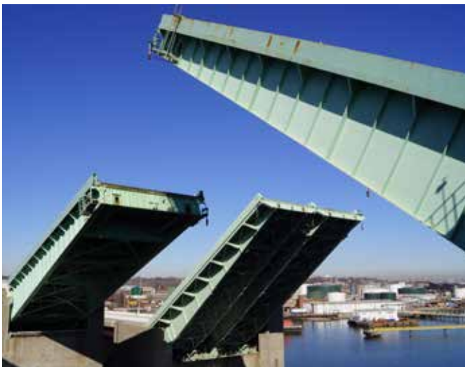
Curtis Creek Drawbridge (I-695)
