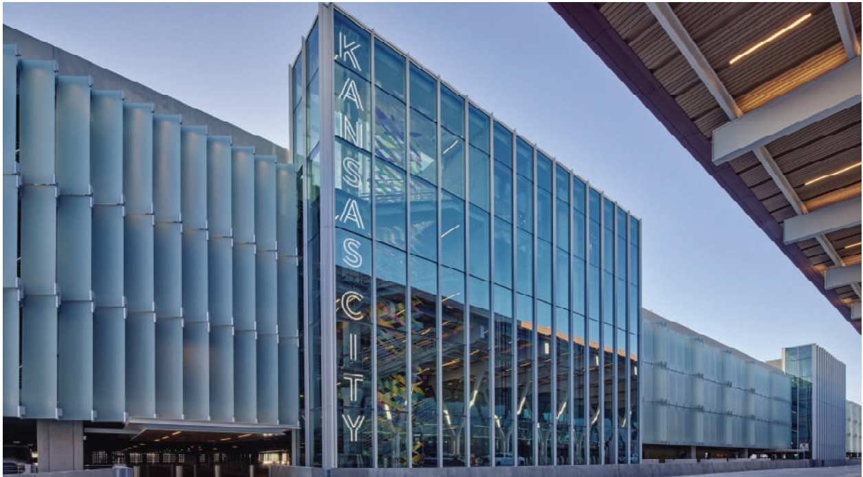
Cover Photo and Above: The Kansas City International Airport New Single Terminal Parking Garage. (Photos courtesy of Trozzolo)
