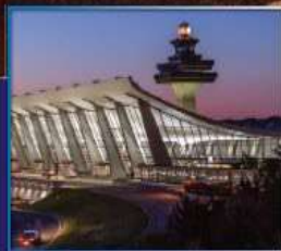
DULLES INTERNATIONAL AIRPORT
