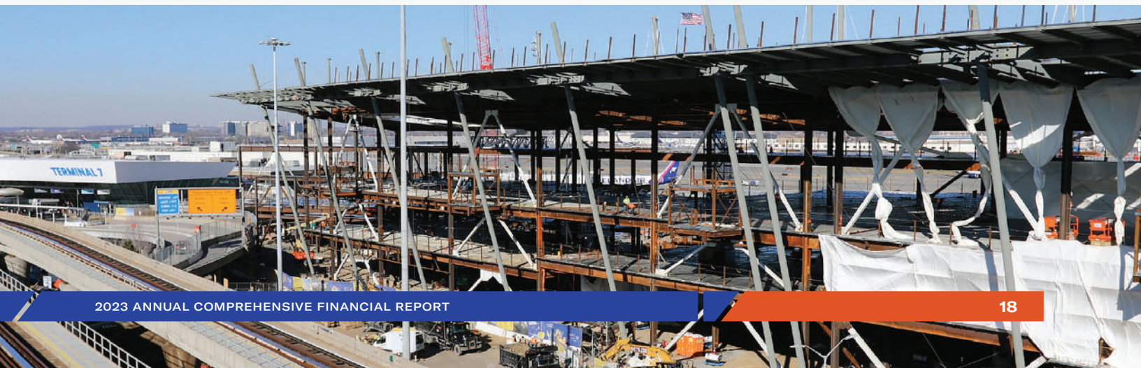
Terminal 6 construction at John F. Kennedy International Airport.
