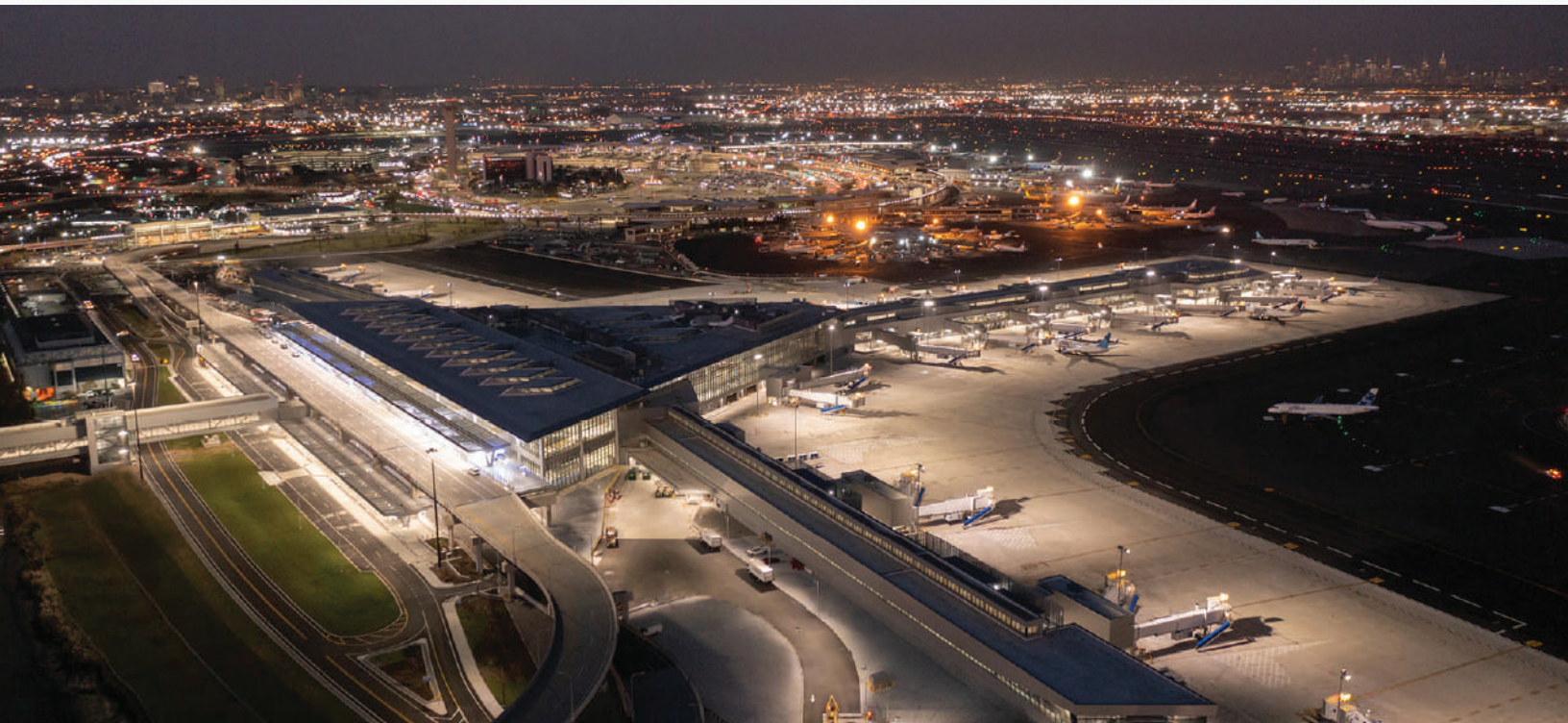
Exterior of the completely renovated Terminal A at Newark Liberty International Airport.
