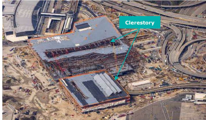
Figure 8-12 Roof Progress up to March 2024
