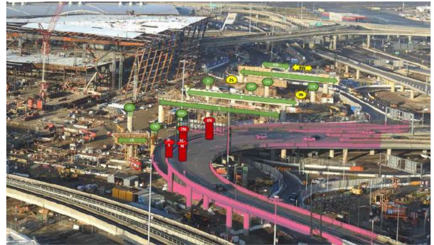
Figure 8-13 T4 Backbone and Roadway Works
