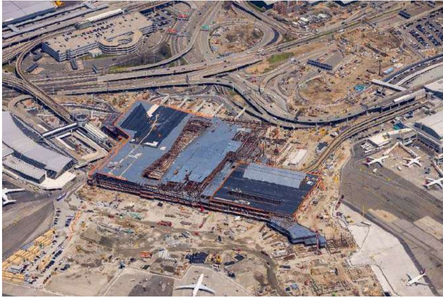
Figure 9-1 Progress on Site up to April 2024
