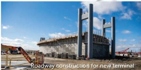
Roadway construction for new terminal
