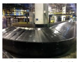
41 LF. For example, if a carousel is 159 LF, the equivalent pier unit would be 159LF/41LF or 3.9 pier equivalents. An airline assigned 4 gates on a LOA would be assigned 4 gates X 0.7 pier or 2.8 pier equivalent or 72% of the carousel.
